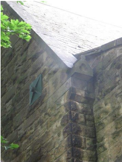
Dampness to the West Elevation from water flowing off of the water table
