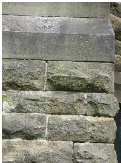
Open joints to South Aisle buttress
