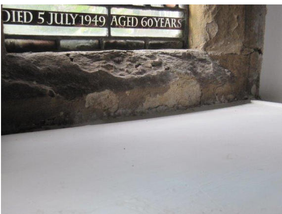
Typical damage to coating to the window surrounds
