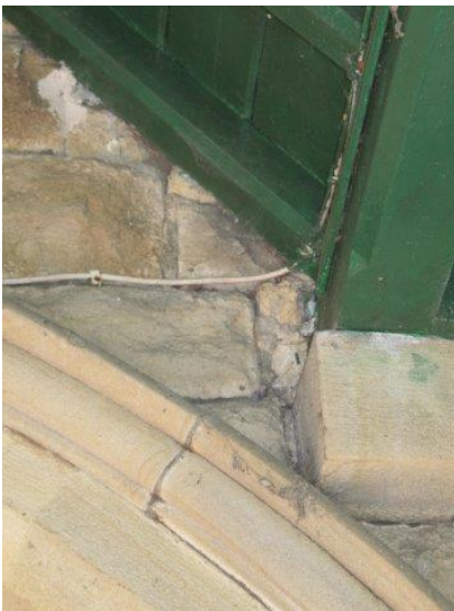
Cracking to North wall of porch over door surround
