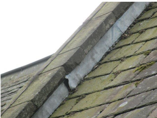
Lifted flashings to North slope of the Nave side
