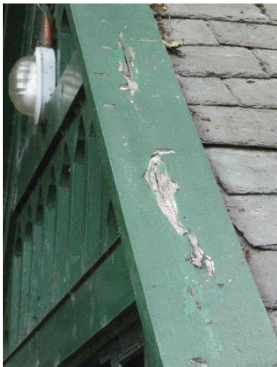
Bare wood and peeling paintwork to porch
