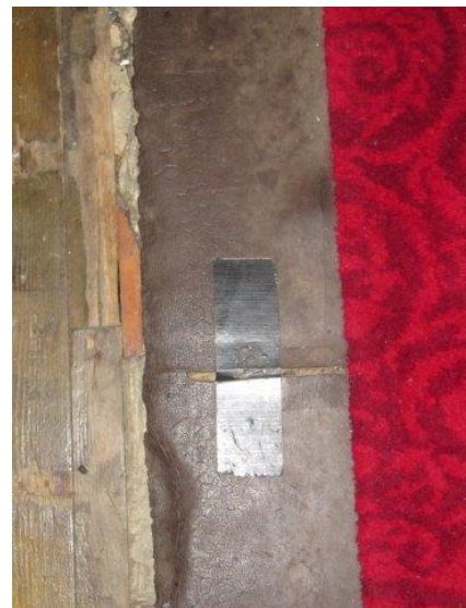
Repaired split to underlay of Nave carpet
