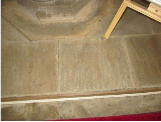
Poor demarcation to change of level near the font
