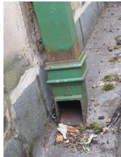
Slipped show to downpipe on North of the Chancel
