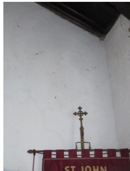
Damage to plaster in the South East corner of the South Aisle
