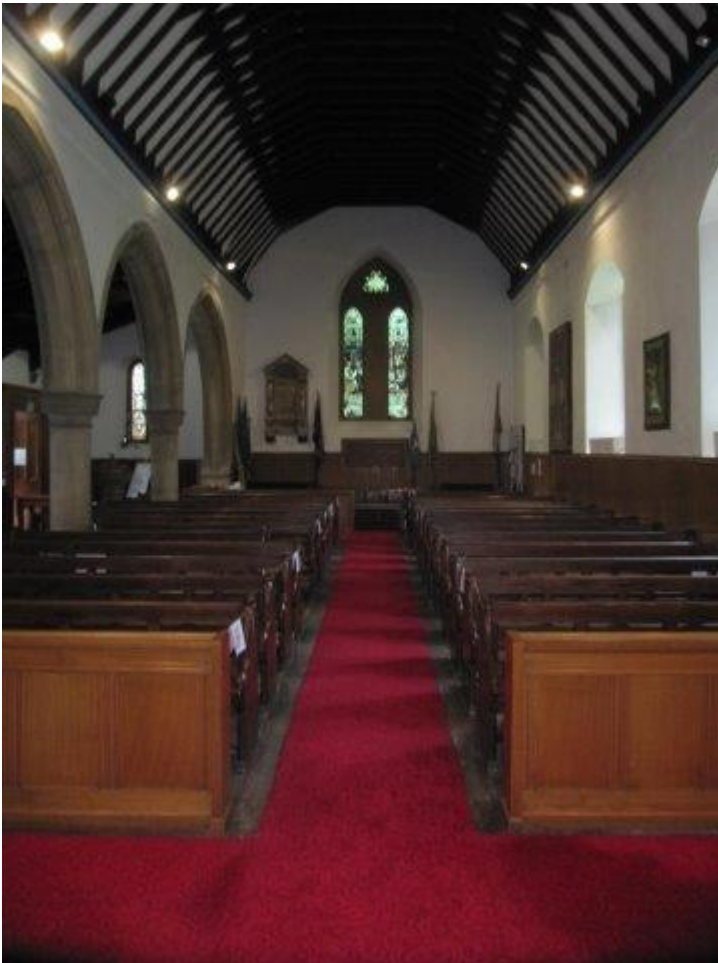
General view of the Nave looking West
