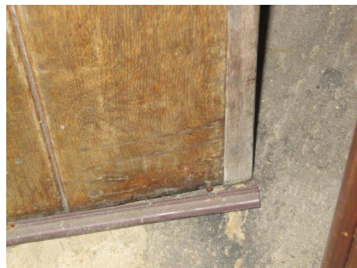
Failing weather / draught strip to base of lobby door
