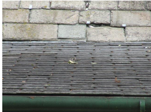
Cracked slate to South slope of the Nave roof (this was noted in the previous report)
