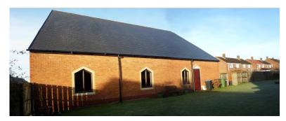
**East Elevation** – Pointed in diagonal cracking at the south east corner at high level. General elevation ok as are the windows though the decoration is beginning to break down on the cills.
