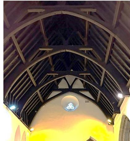
Figure 18– North aisle roof structure
