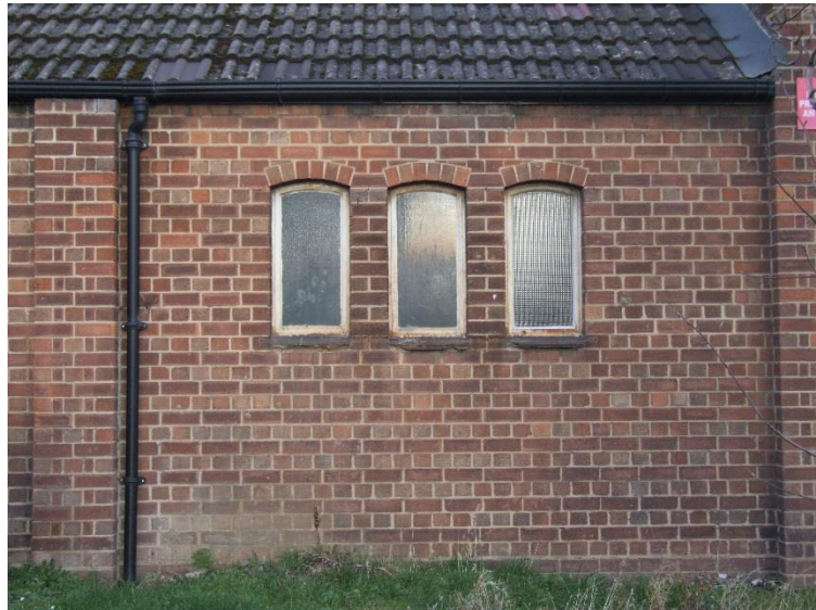
South elevation, damaged plain tile sills; corroded steel windows
