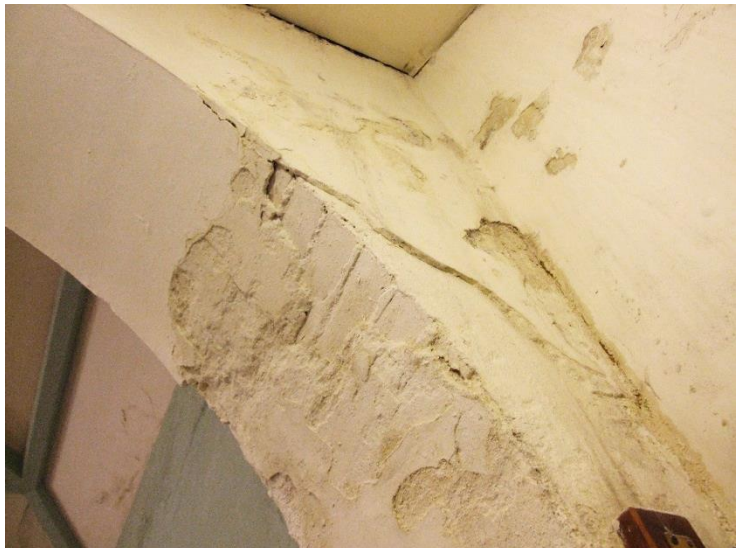
Damp penetration and plaster loss, sanctuary south aisle
