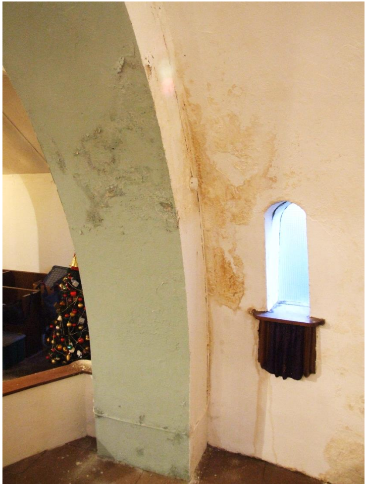
Damp penetration, sanctuary arch, north side detail
