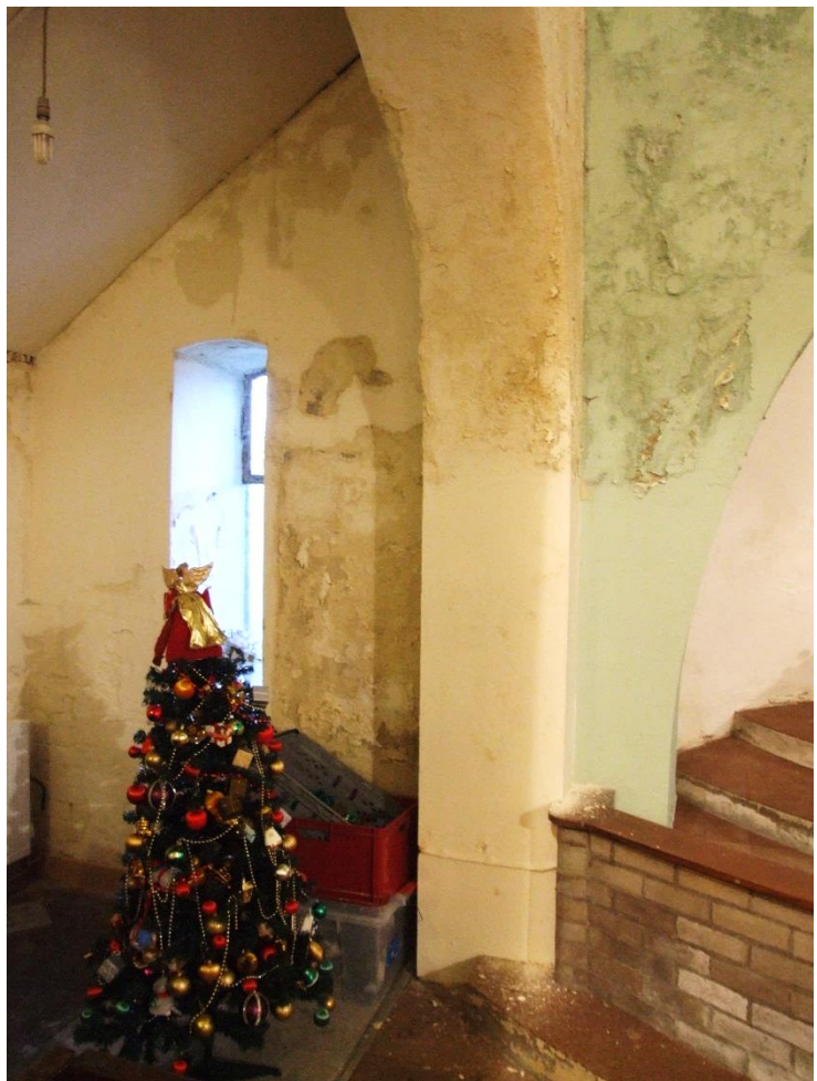
Damp penetration, north aisle, east end
