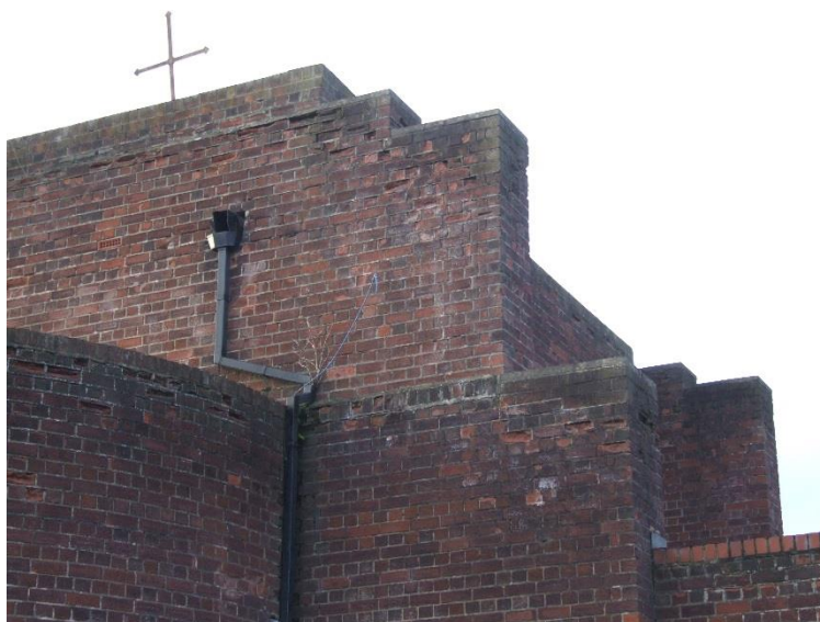
Detail of brick spalling, north east corner
