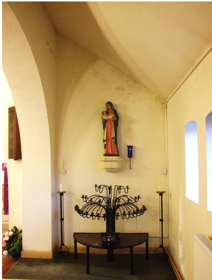
Alcove, south aisle showing high level damp penetration
