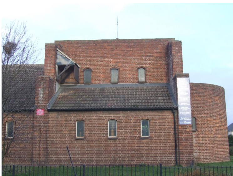
South elevation, chancel area Redundant bellcote
