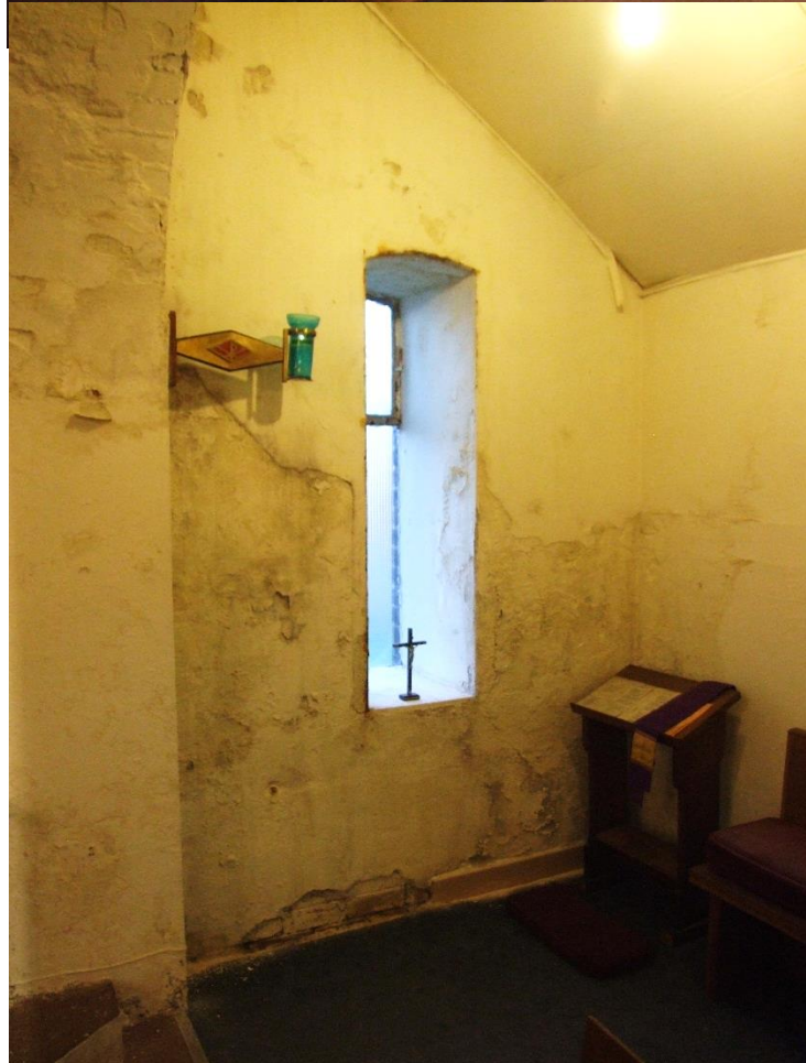
Damp penetration, south aisle, east end of chancel
