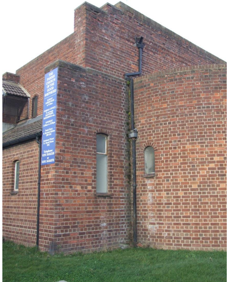
Southeast corner, damage from downpipe leakage
