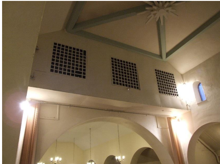
High level, west end of chancel: Organ pipework location, also showing folding screen replacing original slide away doors
