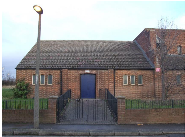
South elevation, main hall (Nave)
