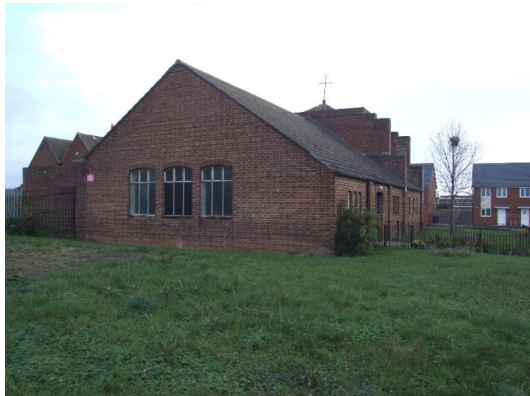
West elevation, main hall (Nave)
