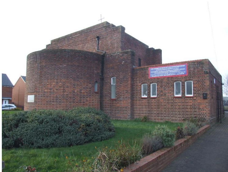
View from northern access route, showing high level brick spalling
