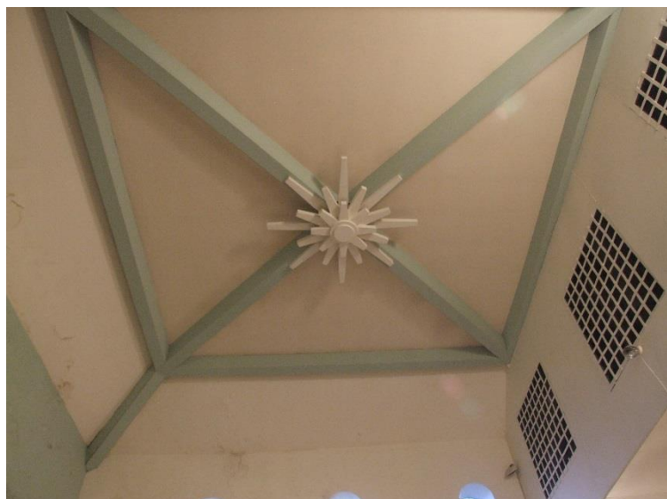
Ceiling detail (chancel), with evidence of damp penetration
