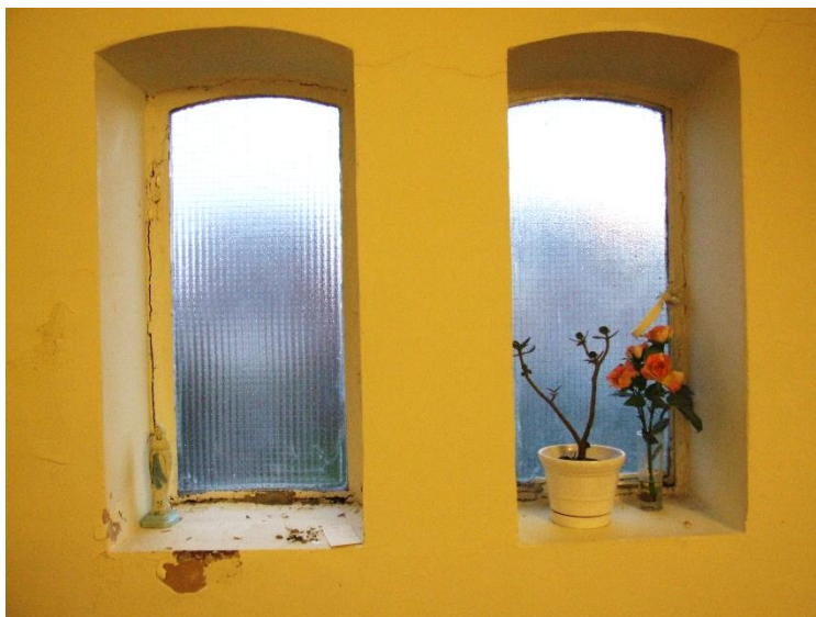
Rusting steel windows in meeting room
