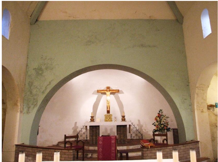
View from chancel to sanctuary showing damp penetration
