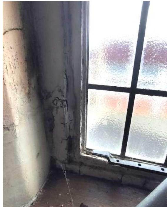
39. Details of rusted window frame
