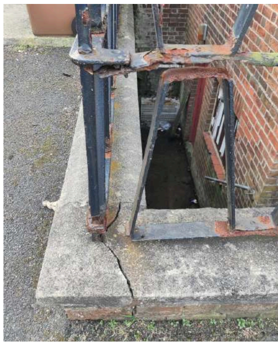
16. Railing and copings in poor condition
