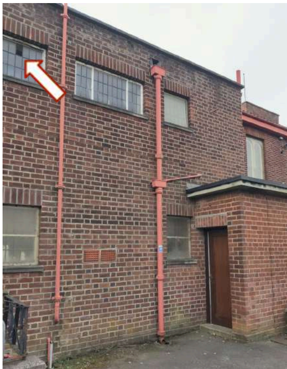
13. Vestry N wall; missing glazing pane (arrow)
