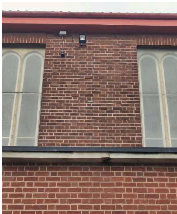
11. Condition of vertical cracking in N wall
