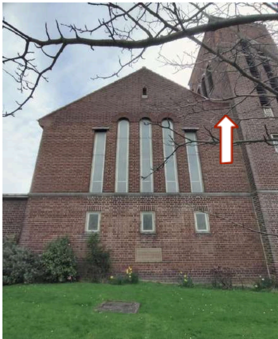
7. W elevation. Water ingress from gutter (arrow)
