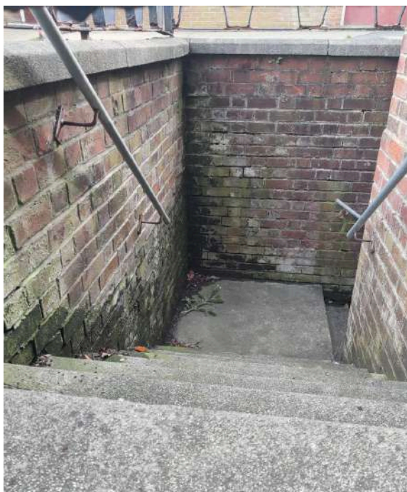
15. Water ingress into retaining wall to basement
