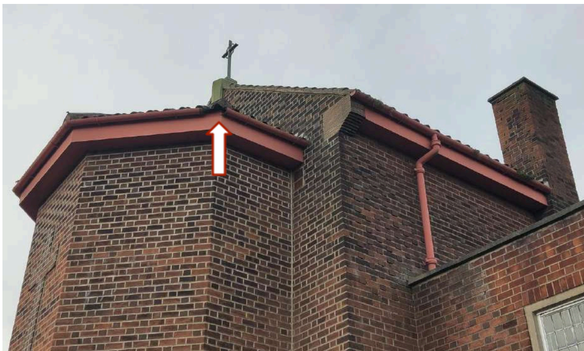
17. Missing gutter to Chancel (arrow); top of chimney needs pointing repairs
