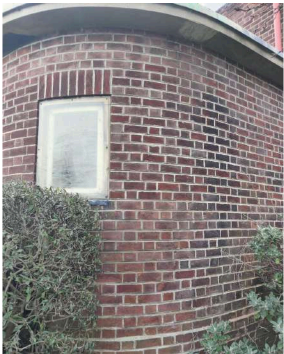
9. Baptistry. Distracting white repointing & past repairs to concrete fascia
