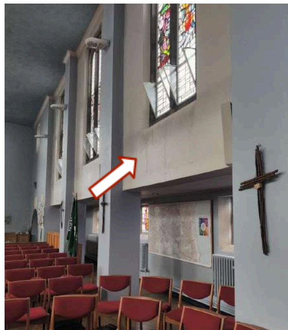
25. N Nave wall. Arrow shows plastered-over original heating outlet positions under windows
