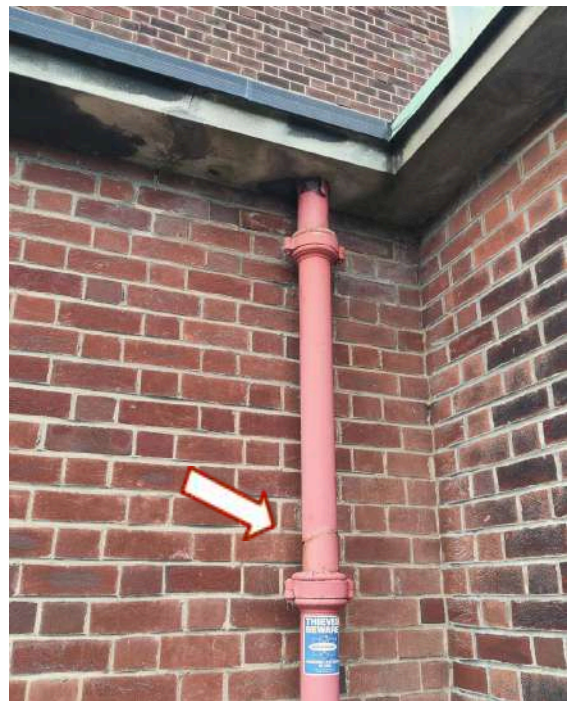
10. Original & neat replacement drip detail at Baptistry/ North Aisle. Cracked pipe (arrow)
