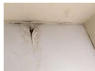
3. Lath and plaster ceiling above Narthex north lobby is water damaged.
