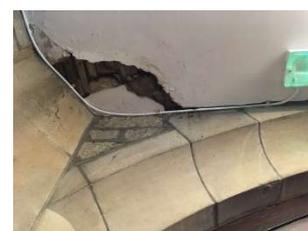
4. Vaulted lath & plaster above Narthex is suffering from water ingress.
