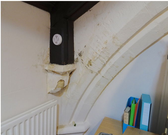
South Aisle first floor – east room south wall damp on arch base
