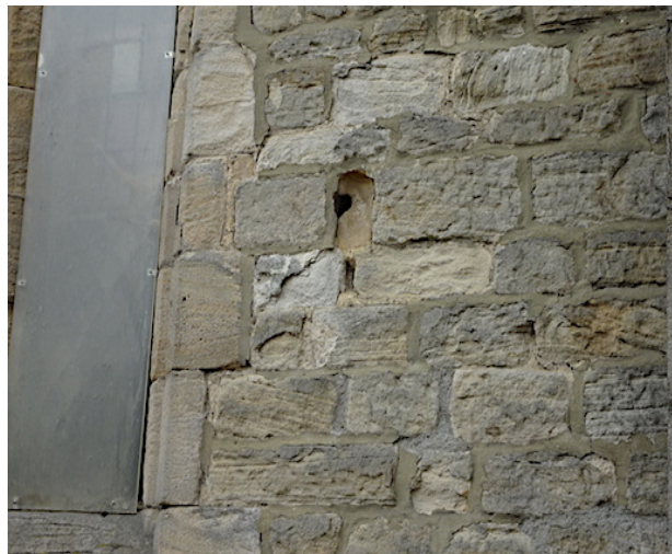
West end South Aisle wall – defective and eroded stonework
