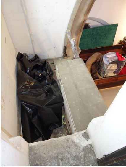
Access landing for Bell Turret at west end
