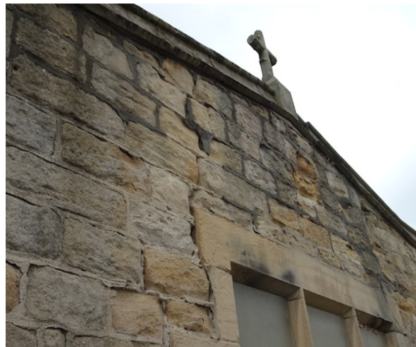
South East Vestry south wall – open joints and badly eroded stone
