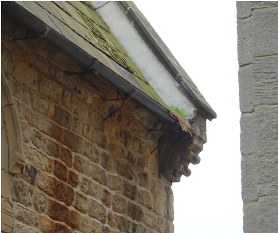
Nave roof, north side, west end – gutter filled with plant life
