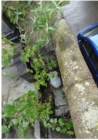
Sump at north end of east gutter
