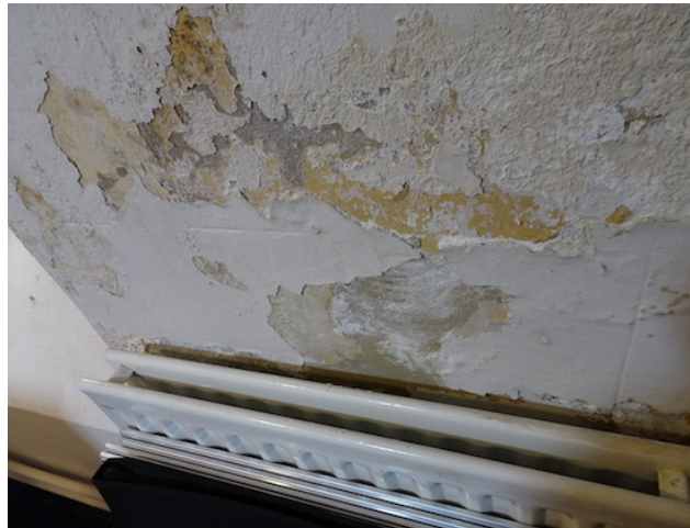
South Aisle first floor – east room showing penetrating damp east wall
