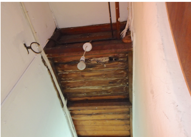
Ceiling of south recess at west end showing rotten boards
