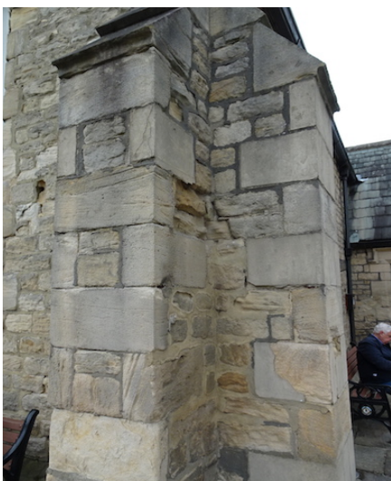
South west end of South Aisle –buttress stonework
