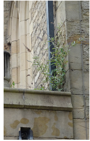
Sump at north end of east gutter
