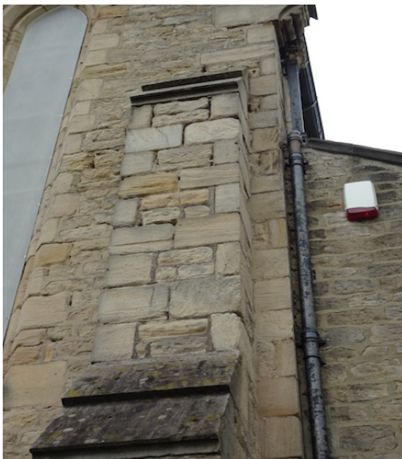
West end Nave wall – south buttress open joints
