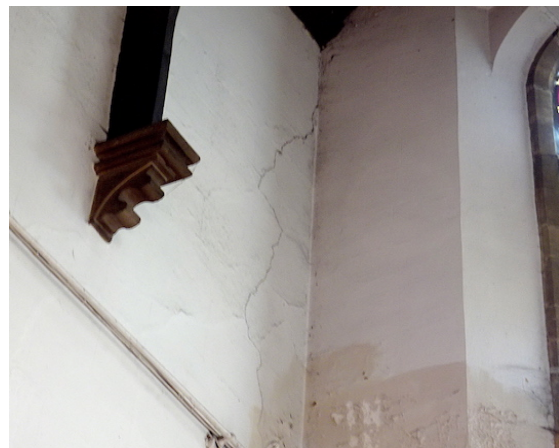
South west corner of Nave showing vertical crack in wall
