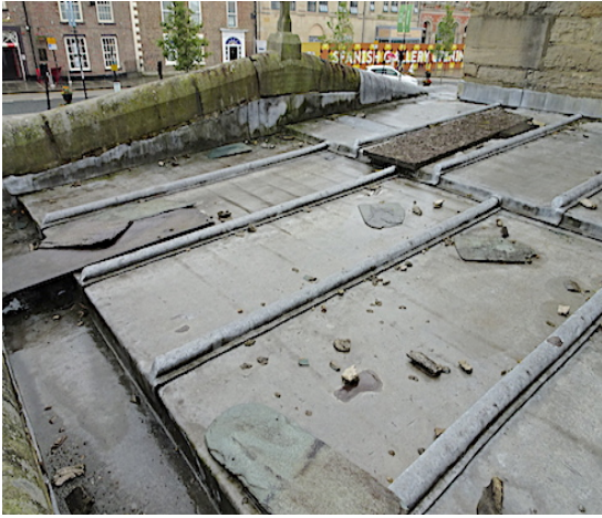
South East Vestry roof – poor condition and defective gable.
