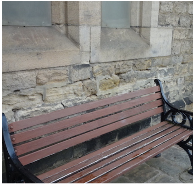
South Aisle wall – eroding stonework below sills and to each window
