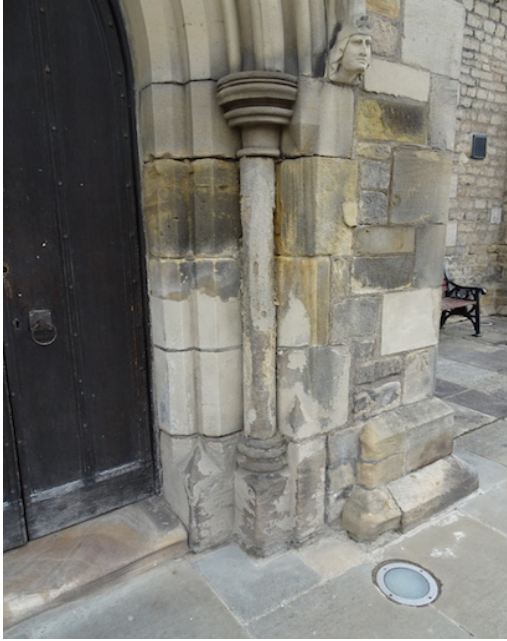
South Porch – eroding stonework to east column and arch
