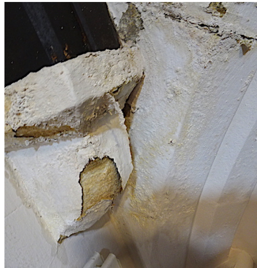
Detail of base of arch
