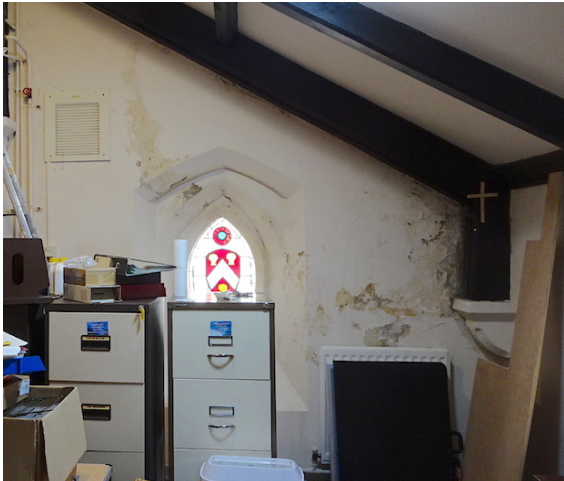
South Aisle first floor – east room showing penetrating damp
