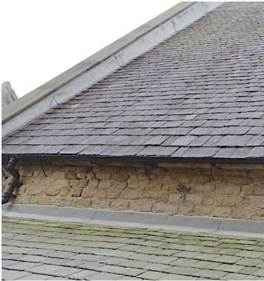
Chancel north side – open joints to north wall.
