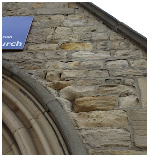
South Porch – stonework to east of entrance arch
