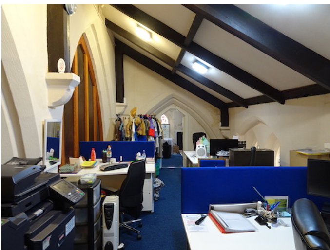
South Aisle first floor – central room leading to east room
