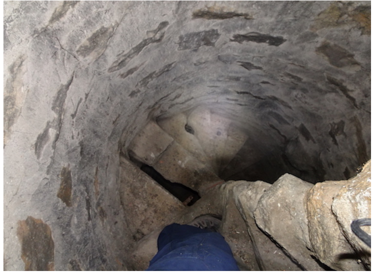
Bell Turret staircase showing missing and defective steps
