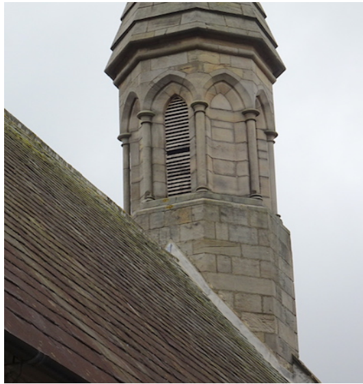
Bell Turret east side – missing timber louvre. (South side also).
