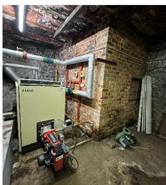
Figure 79 – boiler with new pump
