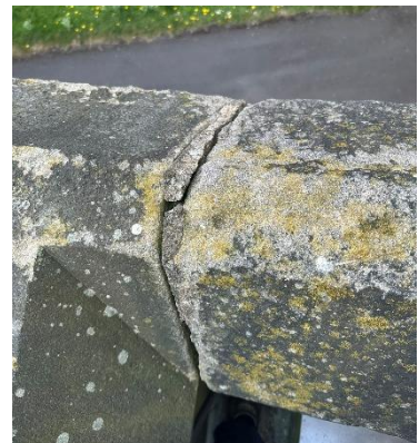
Figure 6 – Open joint to SW corner
