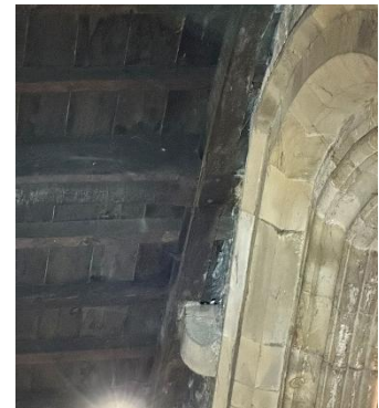
Figure 69 – Arcade wall plate
