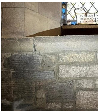
Figure 70 – W wall cill crack
