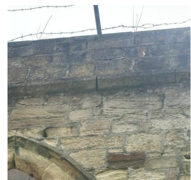
Figure 29 – N parapet open joints
