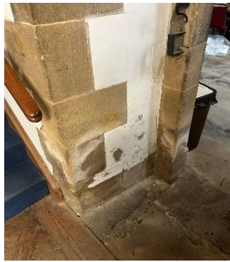
Figure 51 – damp at door
