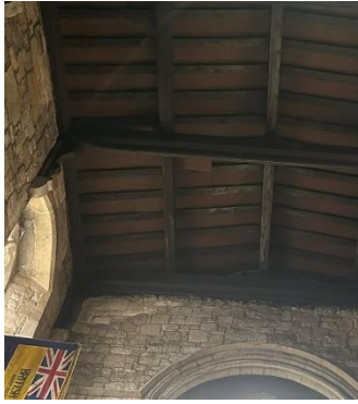
Figure 73 – ceiling board loose
