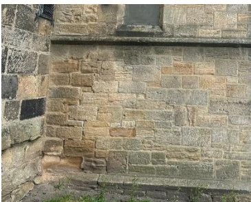
Figure 13 – West cill and erosion
