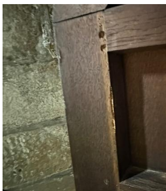
Figure 49 – door woodworm
