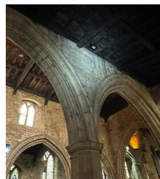
Figure 66 – arcade staining
