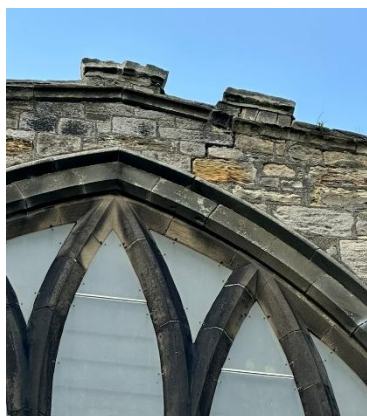
Figure 24 – E crack at window head
