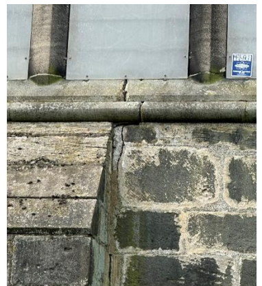
Figure 26 – E gable cill cracking
