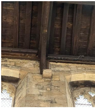
Figure 61 – corbel alignment
