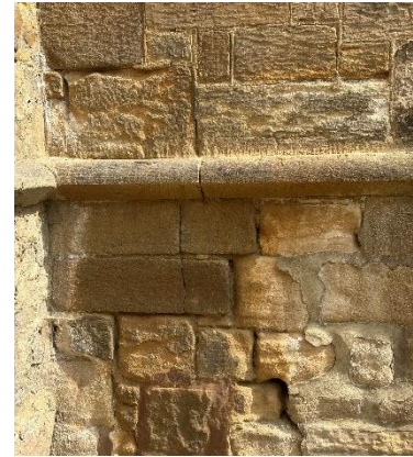
Figure 19 – Crack below string course
