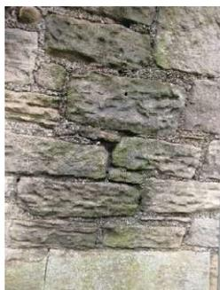
S Transept - open joints between hopper and top of buttress.
