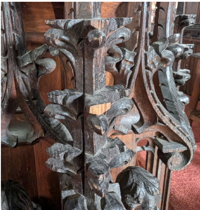
Minor mechanical damage to decorative timber.
