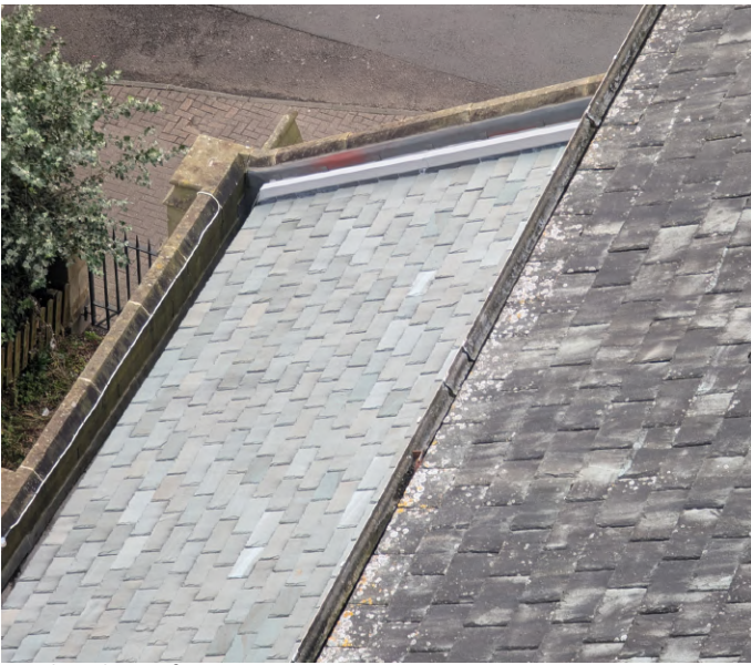
South Aisle Roof - new in 2022
