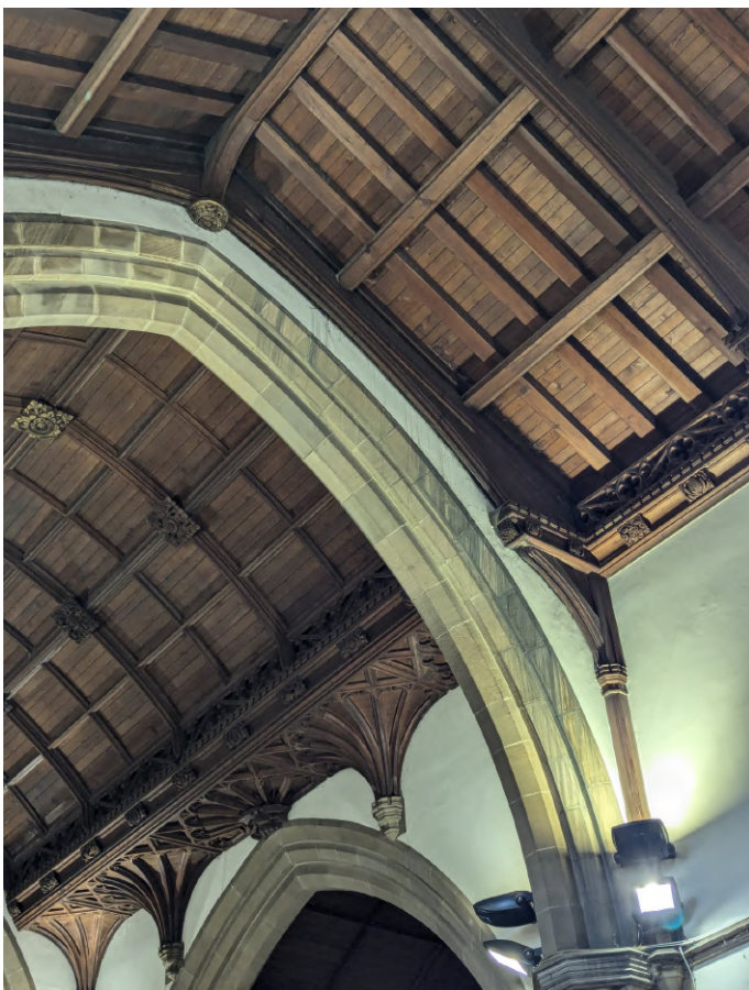
Suspended timber ceilings to nave and chancel. Chancel arch to centre.
