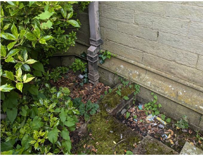
Ensure gulleys are clear and free-flowing.
