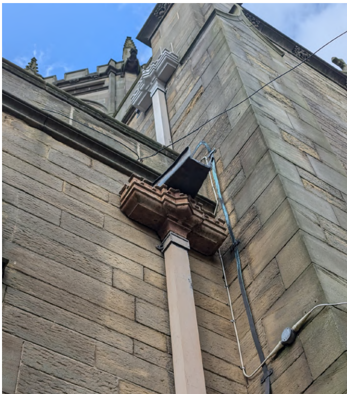
Hopper at south aisle with refurbished hopper of the west side of the north transept (refurbished 2022).
