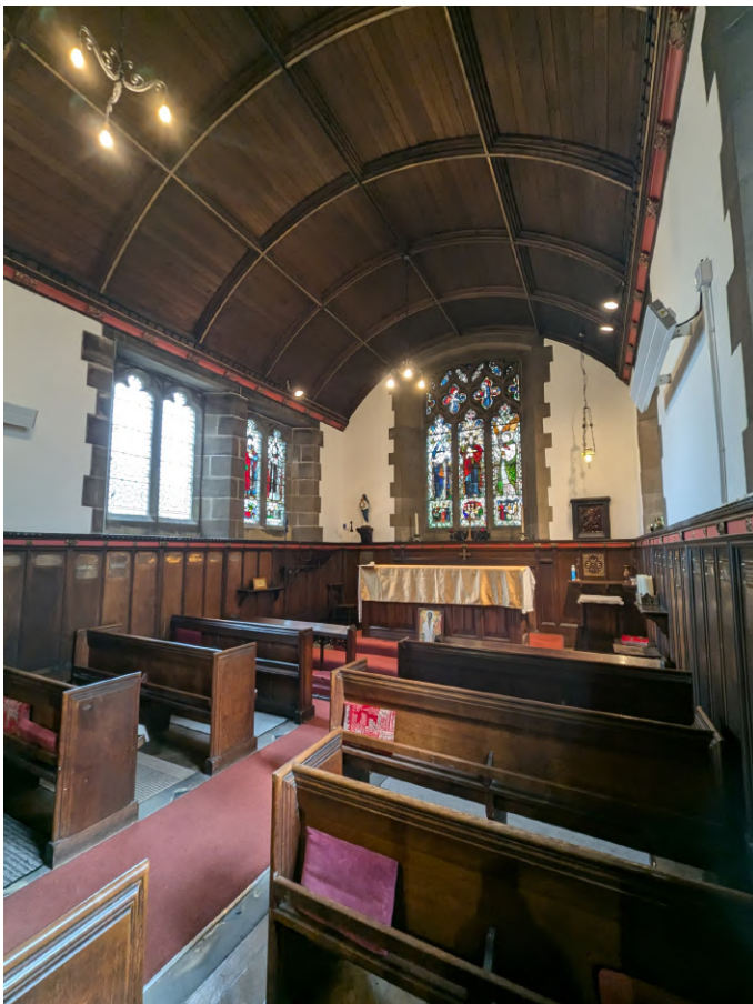
Retro-chapel. New infrared heaters installed.
