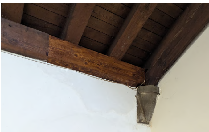
Repairs to previous area of water ingress to south aisle.
