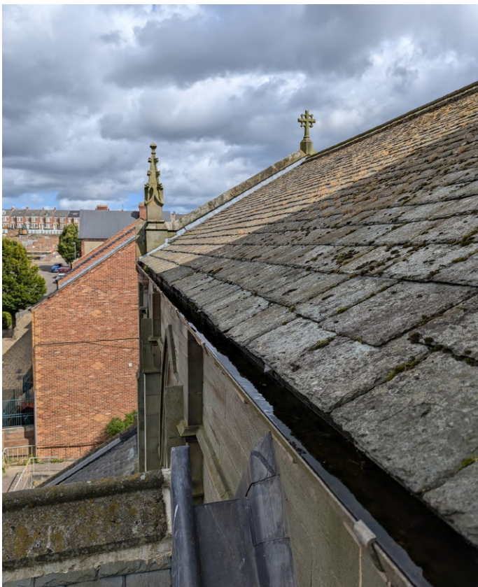
North Chancel Roof - gutter recently cleared, in fair condition
