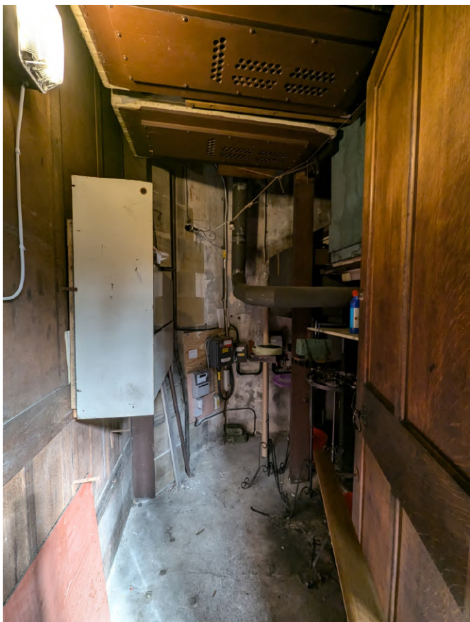
Room below organ chamber.
