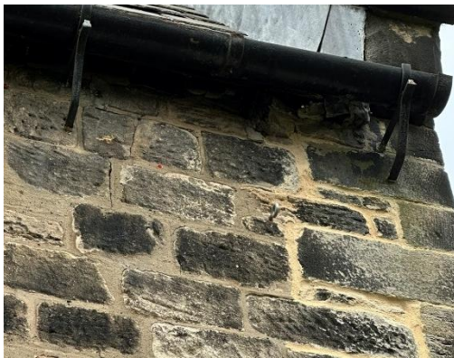
Figure 8 - South Chancel crack near wall plug & new pointing
