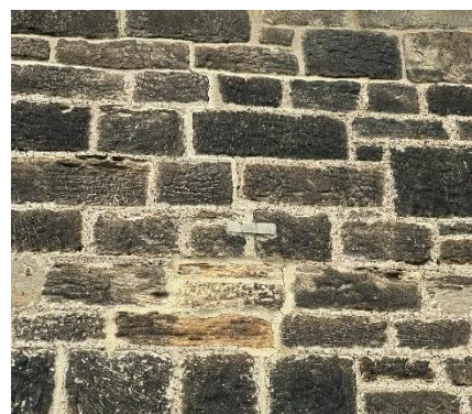
Figure 6 - Crack monitor at S Nave
