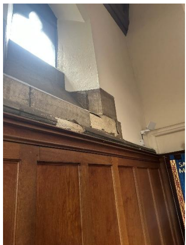
Figure 22 – Chancel stone damage
