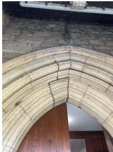
Figure 12 - movement to porch arch
